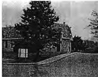
2) FTH – Exterior View
