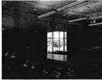
14) TPL – Interior View
