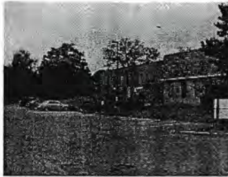
1) FTH – Exterior View
