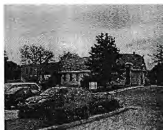
11) FTH – Parking / Exterior View
