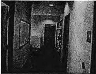
25) TPL – Interior View
